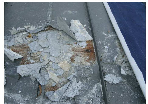
Result of using a hybrid roof
